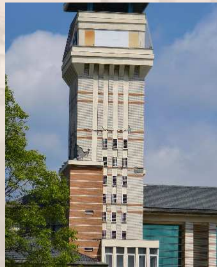
Concrete blocks dropped from tower walls.
